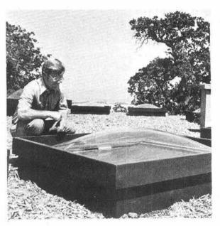
SKYLIGHTS on earth-covered roof provide light for Pete and his family in those portions of the house underground. They also allow for rapid ventilation and are part of a passive solar energy system.
